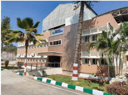
BIMSTEC Centre for Energy Bengaluru, India
